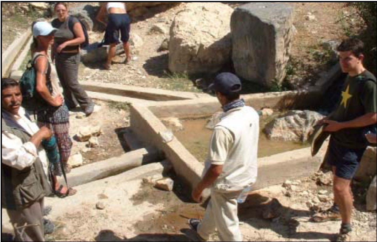
Fig. E20: Channel irrigation system for fruit trees, Dana, west central. Jordan
